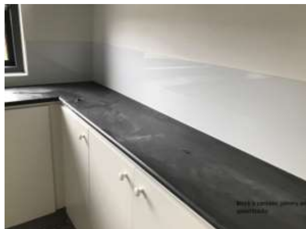
Block B – Multipurpose Kitchen Joinery
