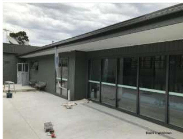
Block C – new windows & entrance
