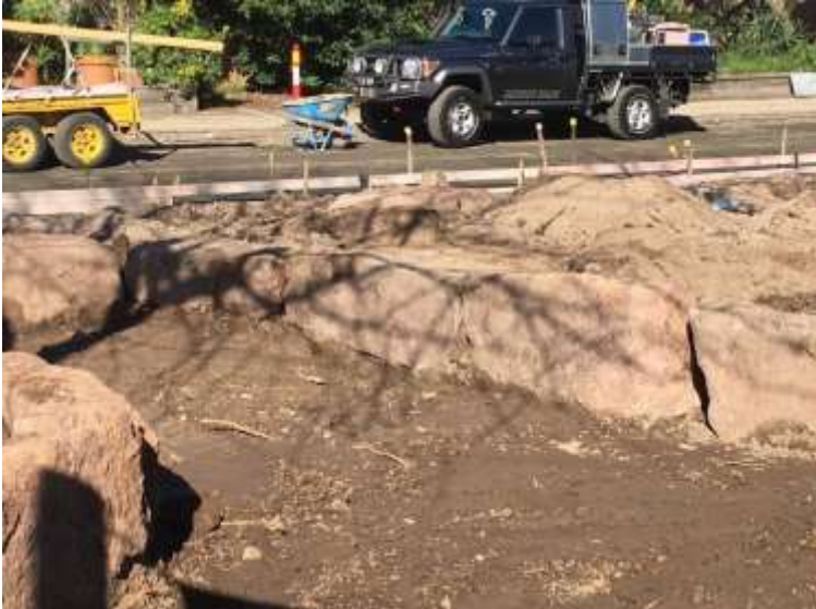
Work continues on the Welcome Garden
