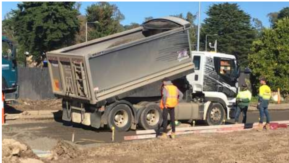
Staff carpark under construction
